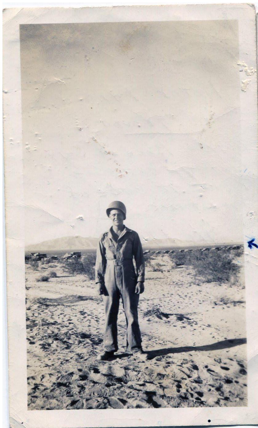
September 6, 1942 "Me. What a sun tan, eh?" Motor park in background (see arrow). Notice piece of Salt flat at extreme right at base of mountains.
