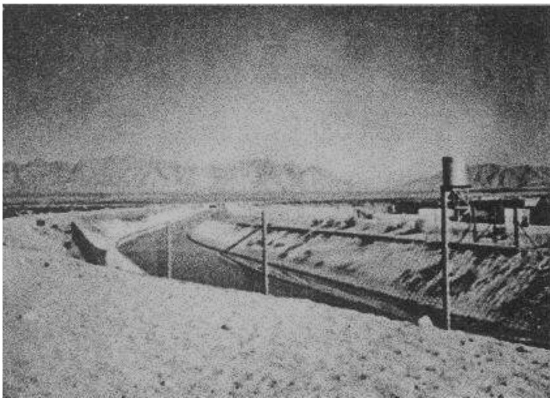
The Aquaduct, Colorado River source, to Los Angeles, over 300 miles away; from a Division History of the California-Arizona Maneuver Area, by Frank Gilchrist, at http://www.90thdivisionassoc.org )
